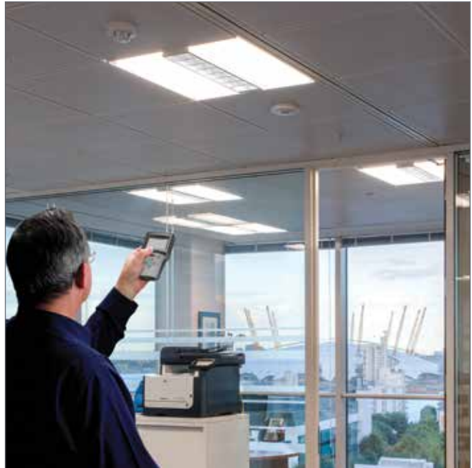
System set-up is carried out using the Infra-Red Master Programmer
