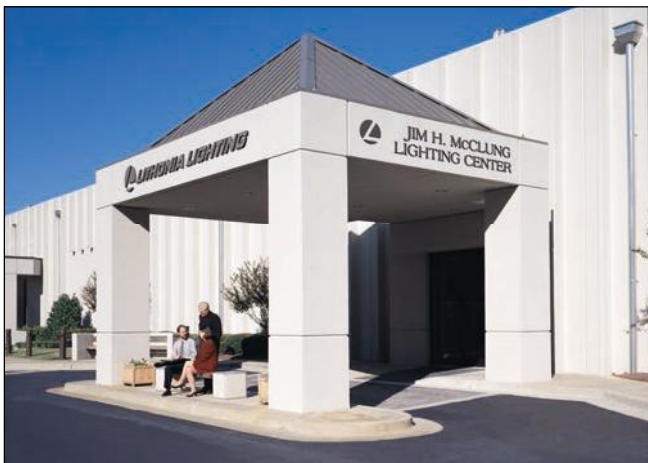
Jim H. McClung Lighting Center, Conyers, Georgia
